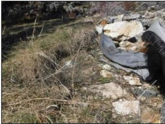
Photo 13. View of erosion along edge of terrace.
