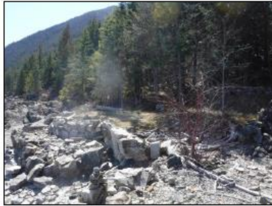
Photo 12. Tiered rock stack retaining walls supporting greenspace terrace.
