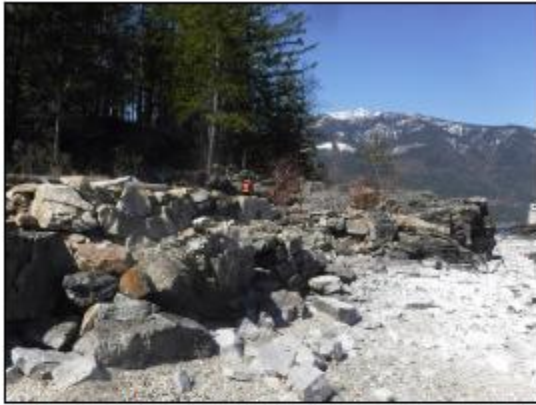
Photo 11. Rugged foreshore with rock retaining walls.
